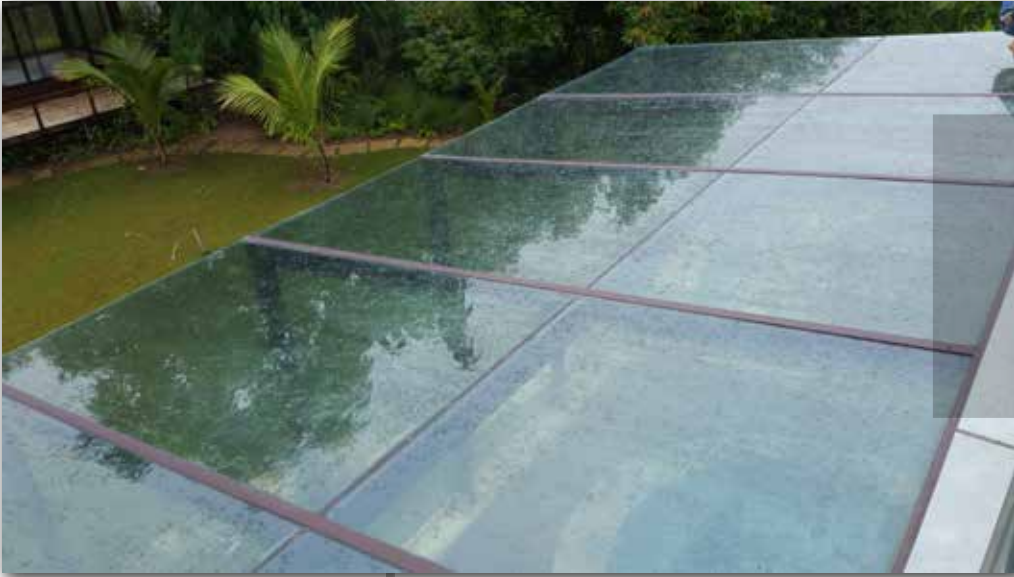
Skylight Mild Steel Frame With Aluminium Composite Panel With Glass
