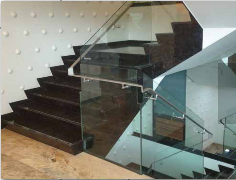
Railing In Stainless Steel Glass On Bolts Chrome Finish
