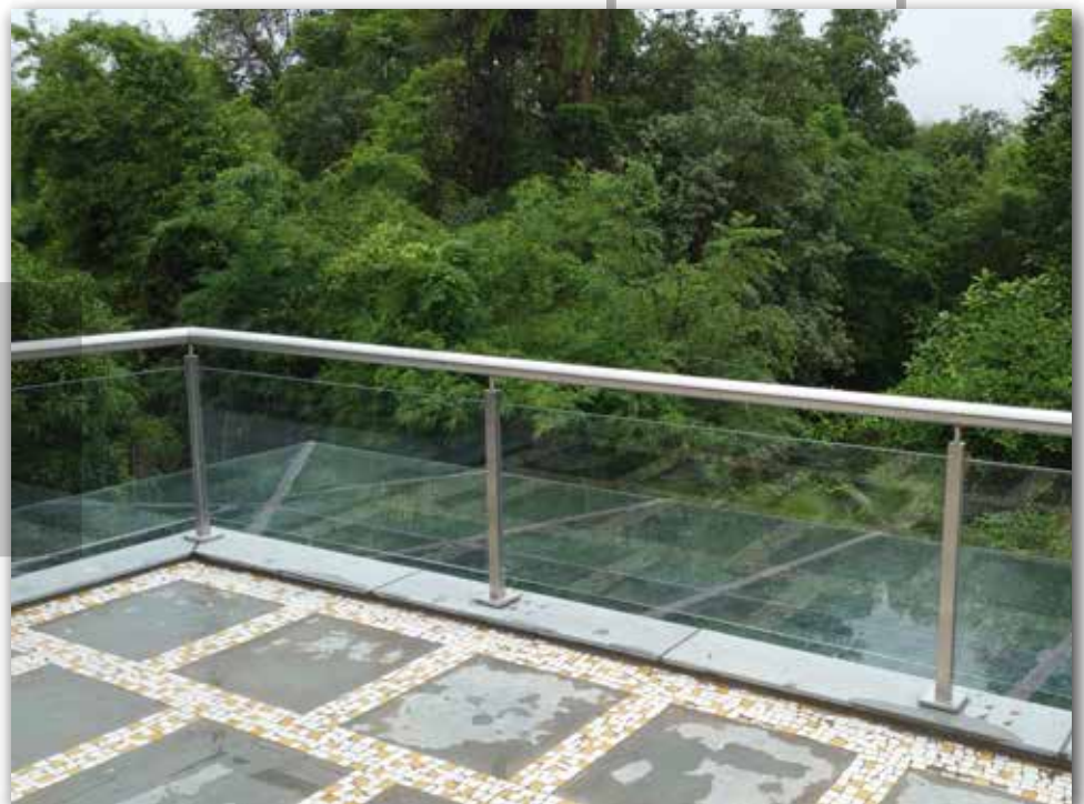
Railing In Glass Baluster In Stainless Steel Chrome Finish
