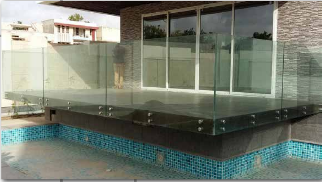
Railing In Glass Glass On Bolts Chrome Finish
