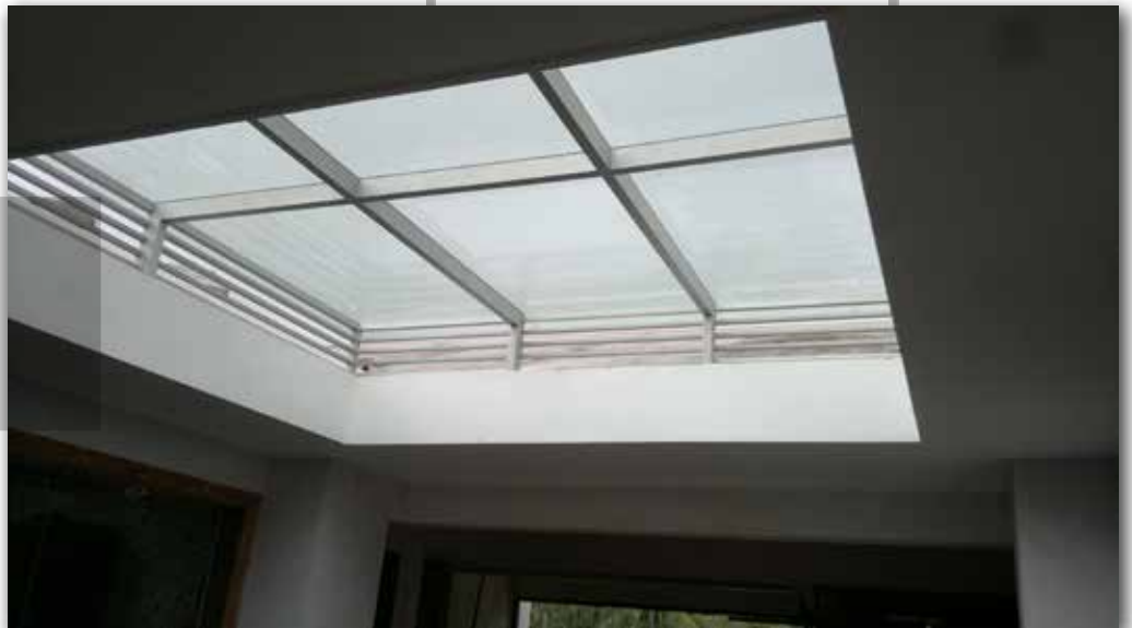
Skylight Aluminium Box Section Frame With Glass
