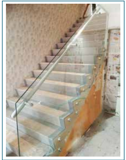
Staircase Railing - Vapi
