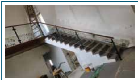
Staircase Railing - Dombivali
