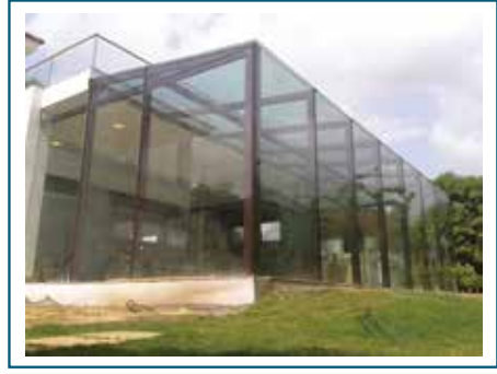
Facade Glazing - Dharampur
