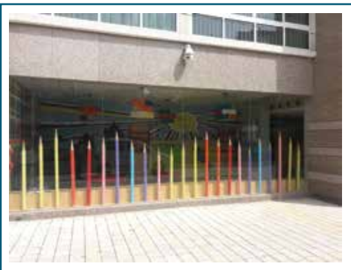
Facade Glazing - Nahar - Borivali
